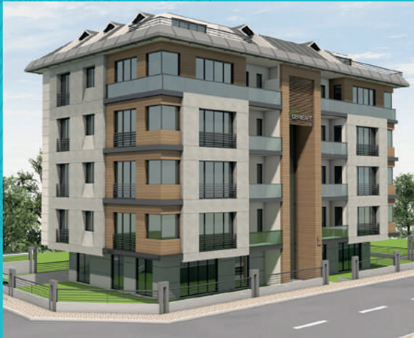
KELES CONSTRUCTION - DEFNE APARTMENT BUILDING - ISTANBUL
