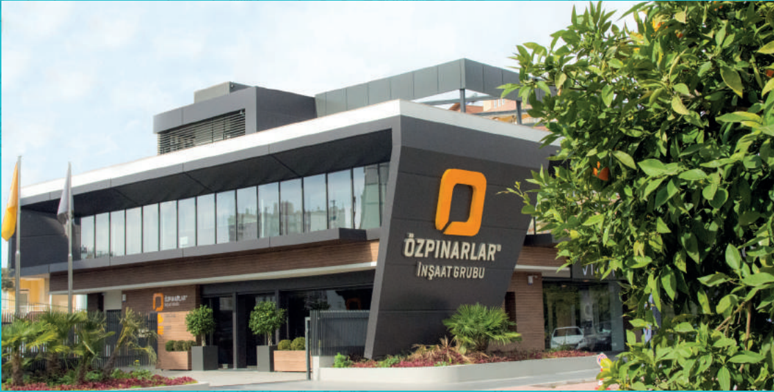
ÖZPINARLAR OFFICE BUILDING - ANTALYA
