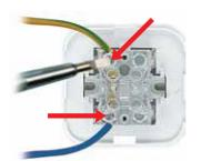
3 Place the connections and tighten the screws
