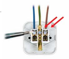
2 Place the connections and tighten the screws
